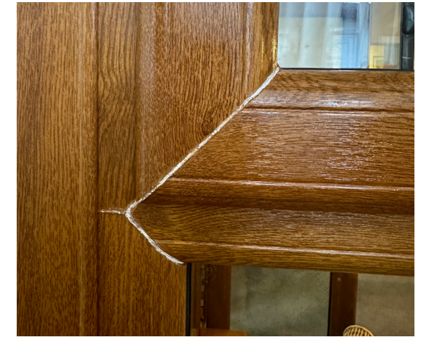
STANDARD CORNER WELD
