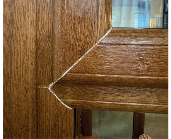
STANDARD CORNER WELD
